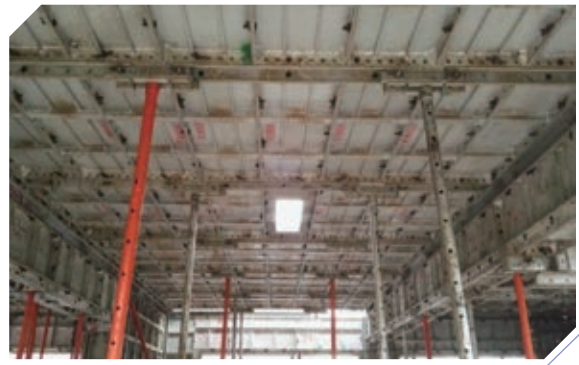
Application of aluminum formwork
