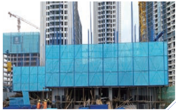
Installation process of climbing frames
