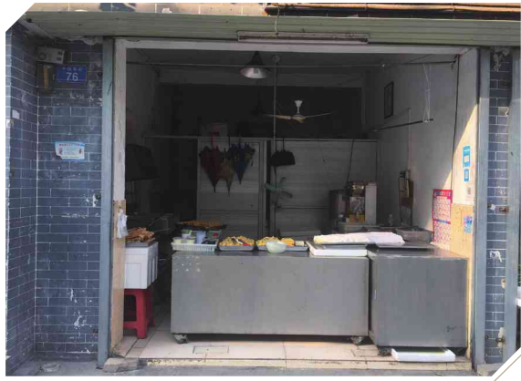
Tofu shop before renovation
